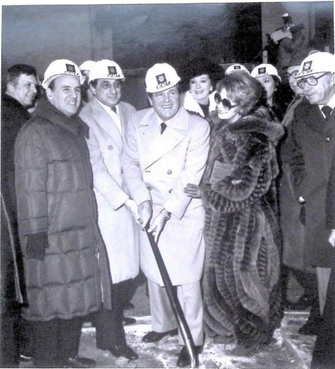
NEW ERA BEGINS - GROUNDBREAKING CEREMONY - DECEMBER 13, 1982.
